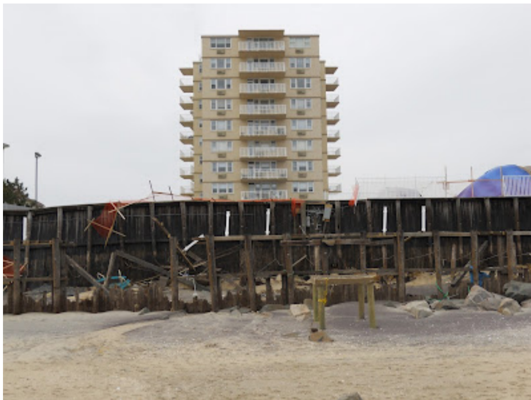
View from beach, four months after Superstorm Sandy
