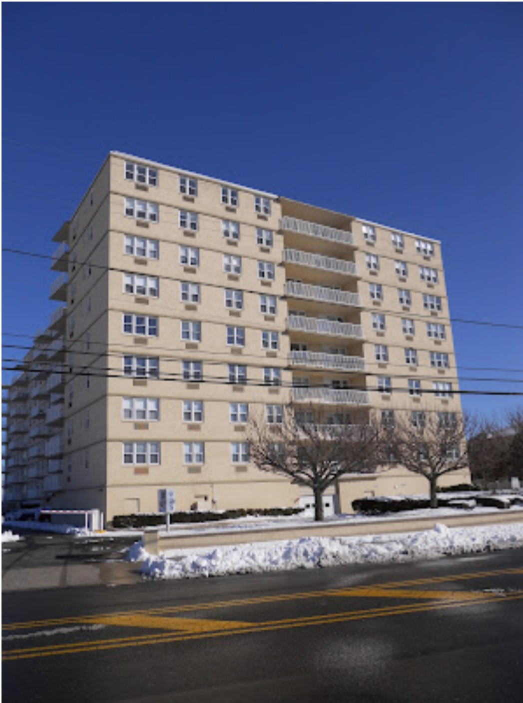
New facade on Harbour Mansion, February 2013
