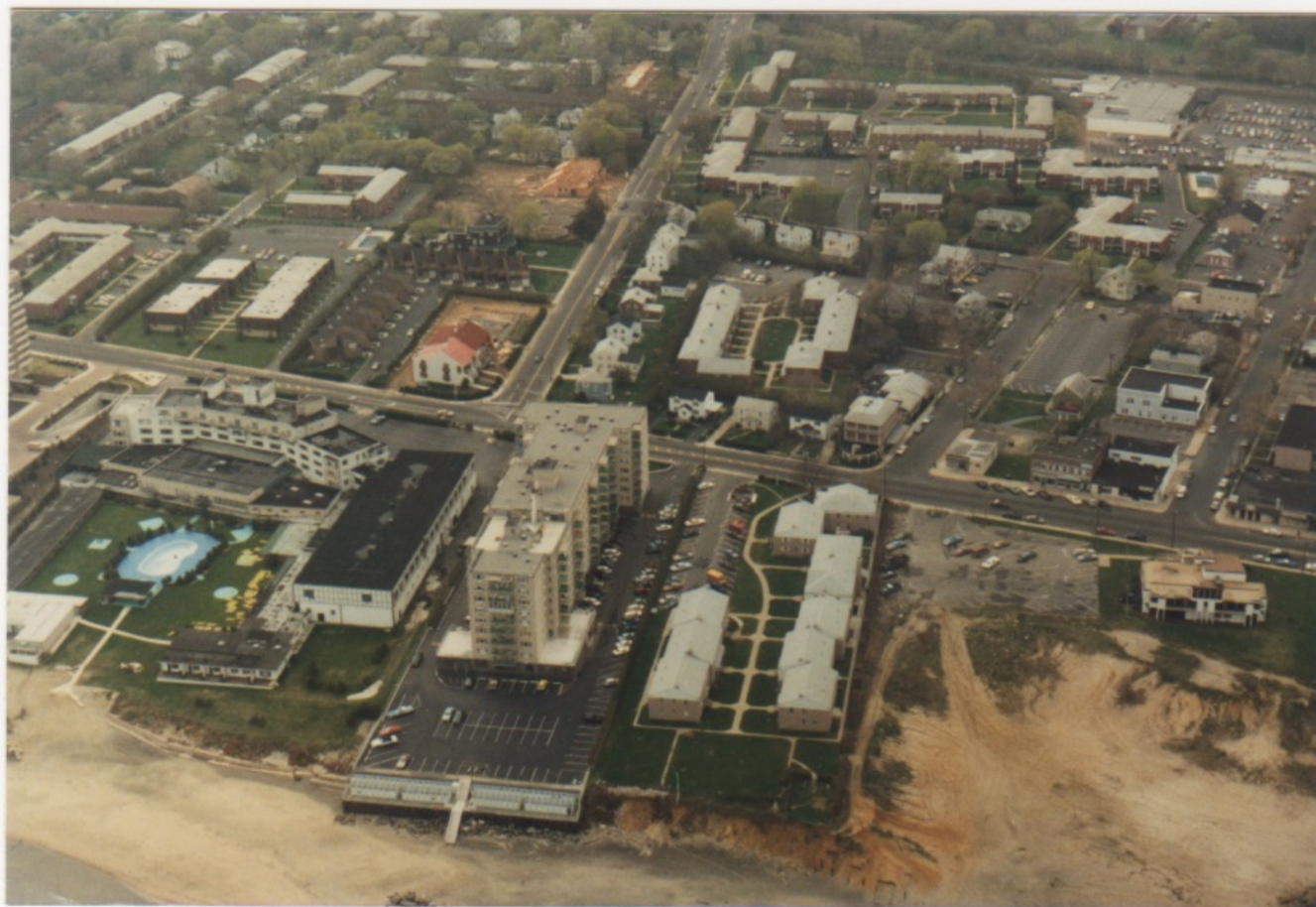
Aerial view of Harbour Mansion (center foreground) with Harbour Island Spa to its left and "big ditch" on the right from early 1980s
