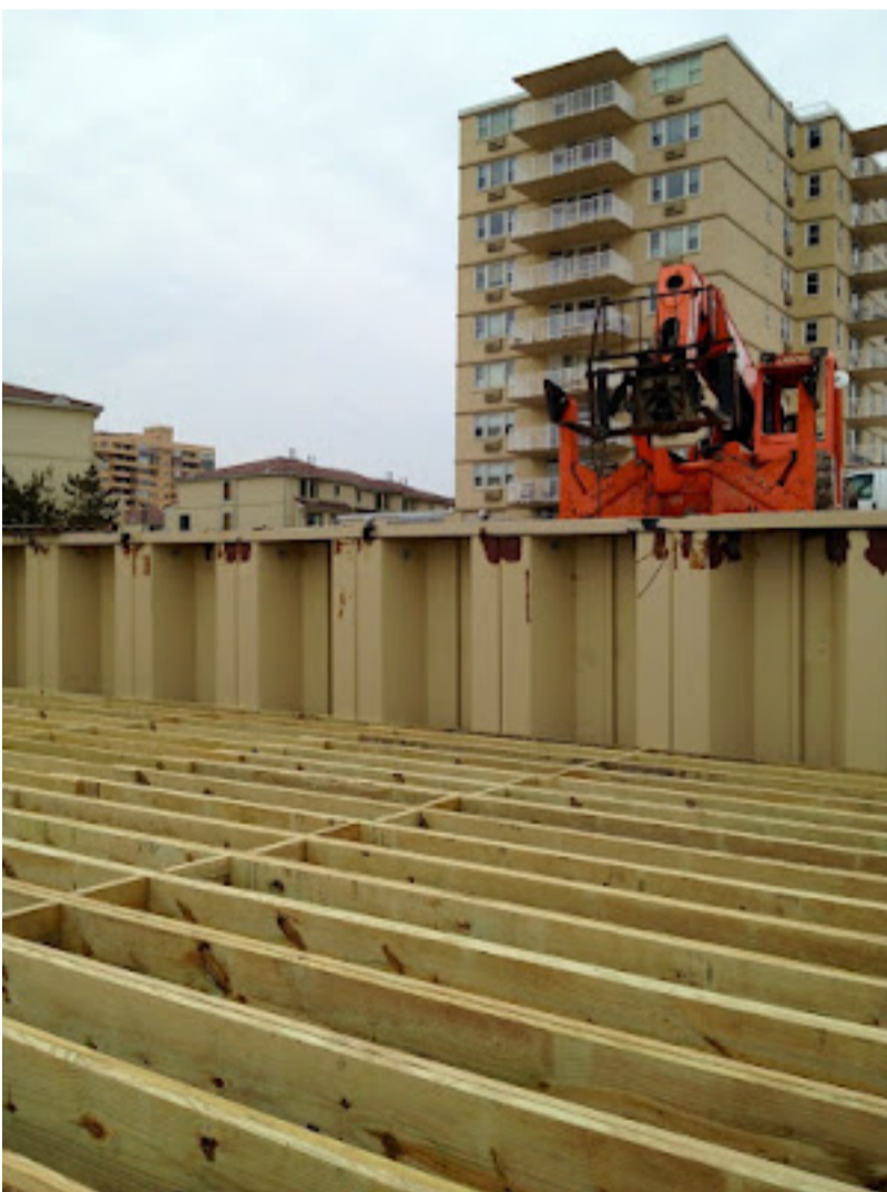
Bulkhead reconstruction, March 2014
