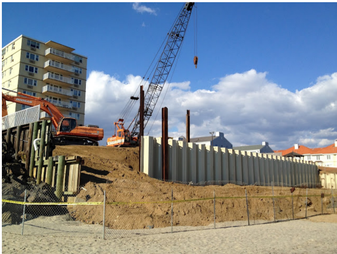
Bulkhead reconstruction, November 2013
